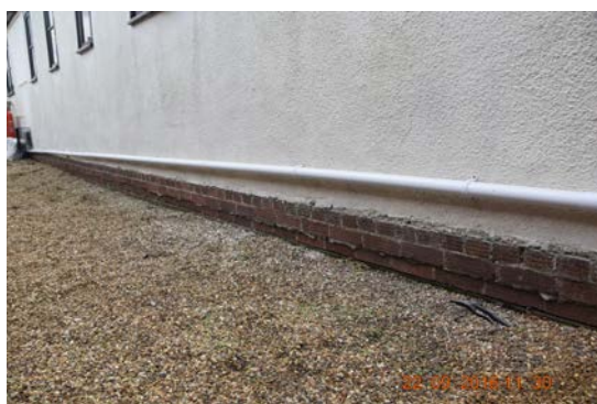
Photo 11 – Upper two courses of low level masonry oversailing rising wall below
