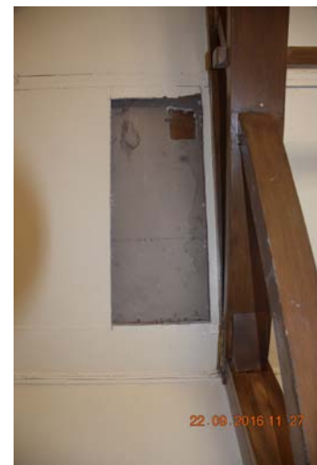
Photo 21 – Section of internal ceiling removed in hall for inspection
