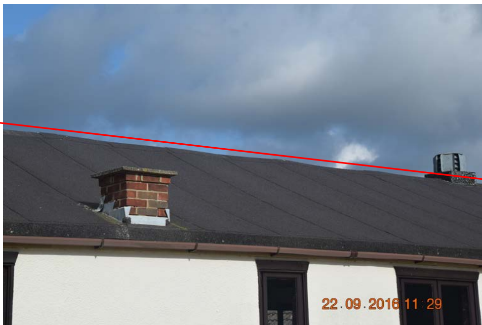
Photo 5 – Undulations in ridge over main hall
