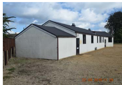
Photo 2 – Photo from the south west showing main hall and store extension
