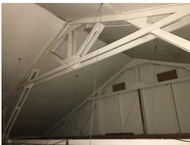
Photo 16 – View of roof structure over bar looking towards the main hall
