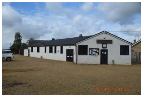
Photo 1 – Front north eastern elevation and eastern gable elevation containing main front entrance door
