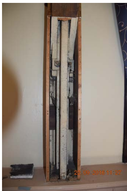
Photo 17 – Column on rear elevation adjacent to the stage
