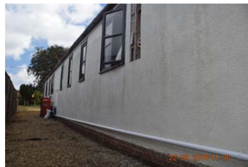
Photo 4 – North western elevation showing low level rising brick plinth
