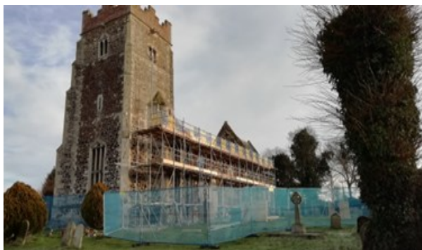
South nave scaffolding - January 2026
